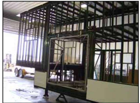
SLIDE OUT CONSTRUCTION IN PROGRESS AT H&H CUSTOM
